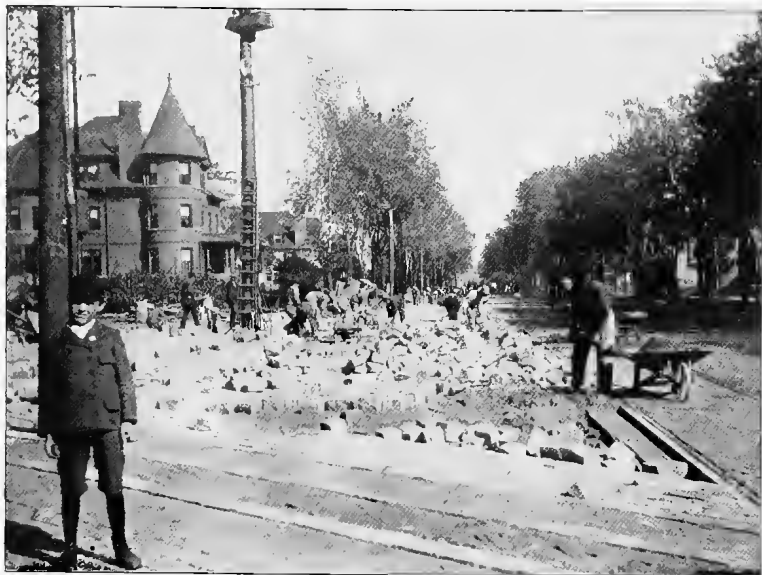
Setting Medina sand-stone blocks on six-inch concrete base covered with one and one-half inches to two inches of sand-cushion.
